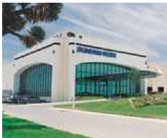
The new Dunham-Bush factory at Nuevo Leon, Apodaco, Mexico.
