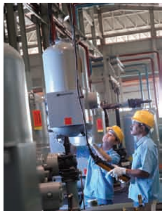
Installing of compressor for water-cooled chiller in Dunham-Bush's manufacturing plant.
