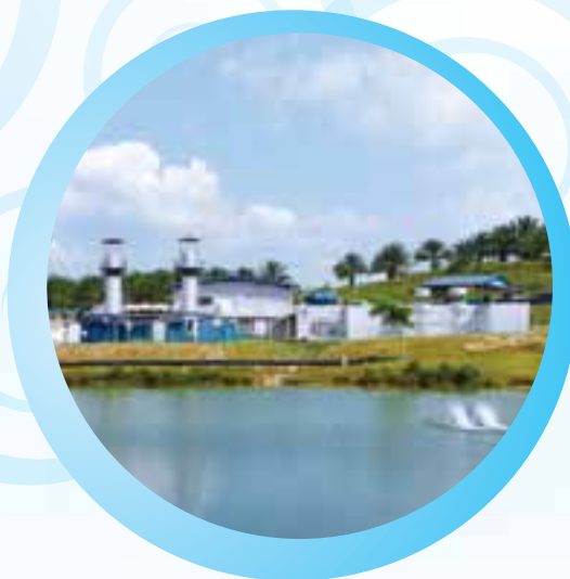
Renewable Energy Centre at Bukit Tagar Sanitary Landfill, Selangor.
