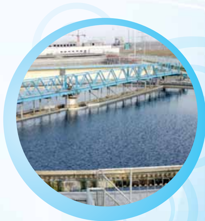
Secondary sedimentation tank - DSG Holdings' water treatment plant in Taian, People's Republic of China.
