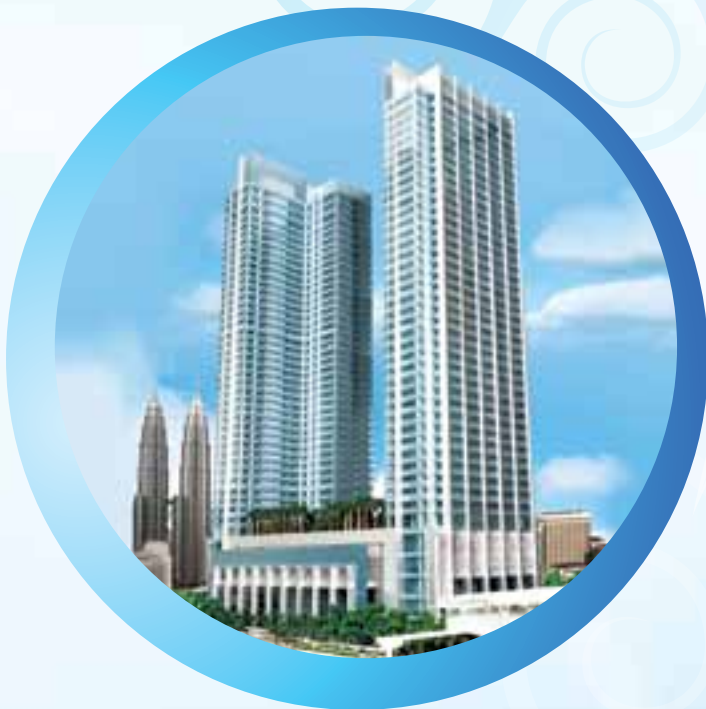
Menara Bangkok Bank @ Berjaya Central Park, Kuala Lumpur.
