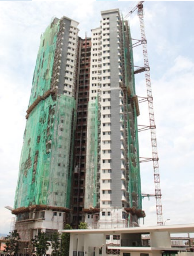
KM1 East, Bukit Jalil, Kuala Lumpur - construction in progress.
