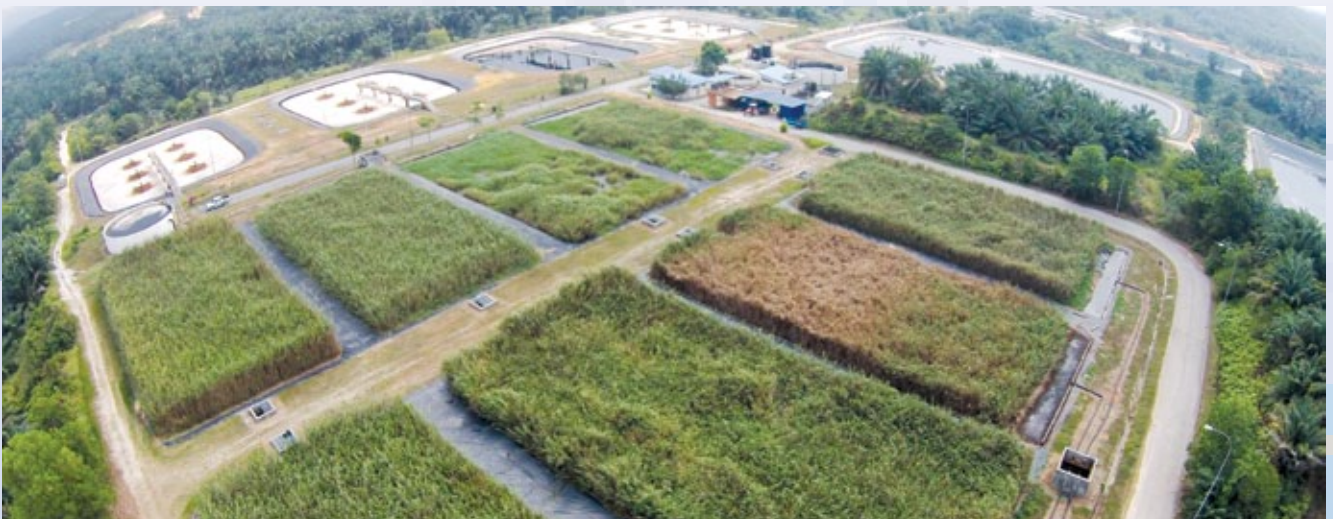
Aerial view of the leachate treatment plant at the Bukit Tagar sanitary landfill, Selangor.
