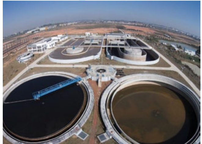
The Jinben Wastewater Treatment Plant in Sanshui District, Foshan City, Guangdong Province, People's Republic of China.
