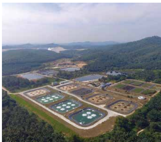
Aerial view of the leachate treatment plant at Bukit Tagar Sanitary Landfill
