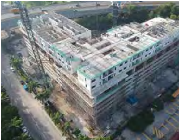
Lanai Residensi - construction in progress
