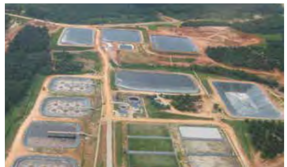
Leachate Treatment System at Bukit Tagar Sanitary Landfill
