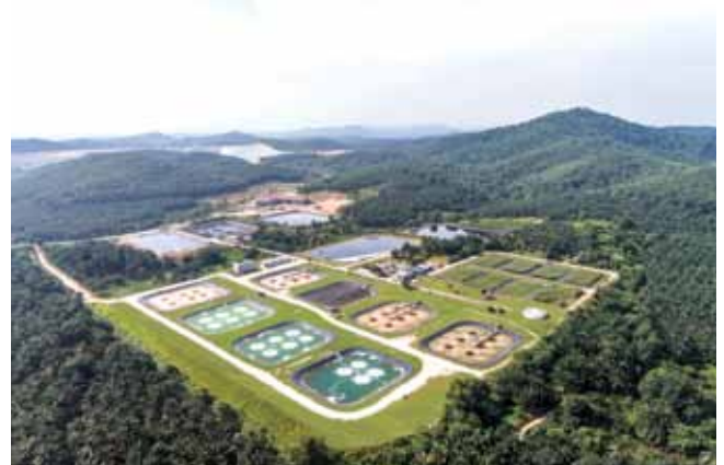
Aerial view of the Leachate Treatment Plant at Bukit Tagar Sanitary Landfill, Selangor.
