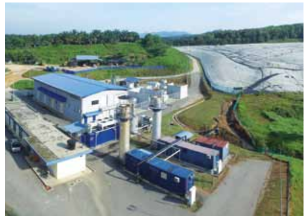
The Renewable Energy Centre at Bukit Tagar Sanitary Landfill, Selangor.
