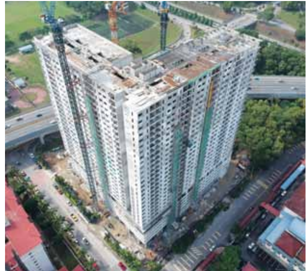
Lanai Residences at Bukit Jalil, Kuala Lumpur - construction in progress.
