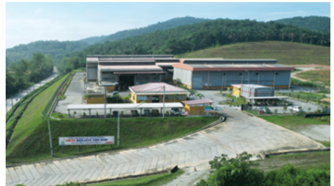
ABSB’s plant at Bukit Tagar, Selangor.
