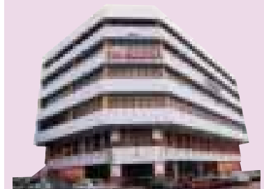
Eng Securities' office building in Johor Bahru.
