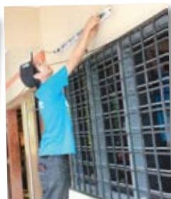
The hotel's maintenance staff repairing the lights of the home.
