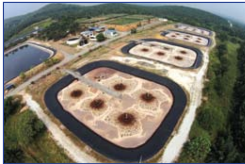
Aerial View of the Leachate Treatment Plant
