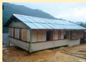
The fully completed 6-module home built by B.Youth volunteers.
