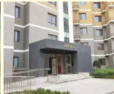
One of the entrances to Block GH, Northern Phase.
