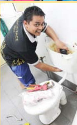
Repairs done by the maintenance team.
