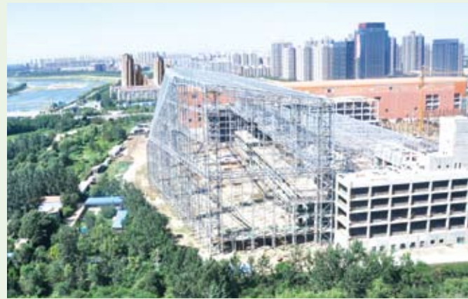
Steel structure of theme park has completed.
