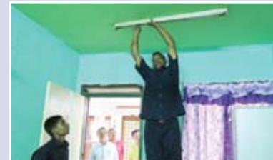
BJGCR's maintenance staff helps to install new lighting for the family.
