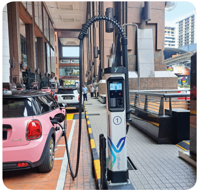
EV Charging Station at Berjaya Times Square
